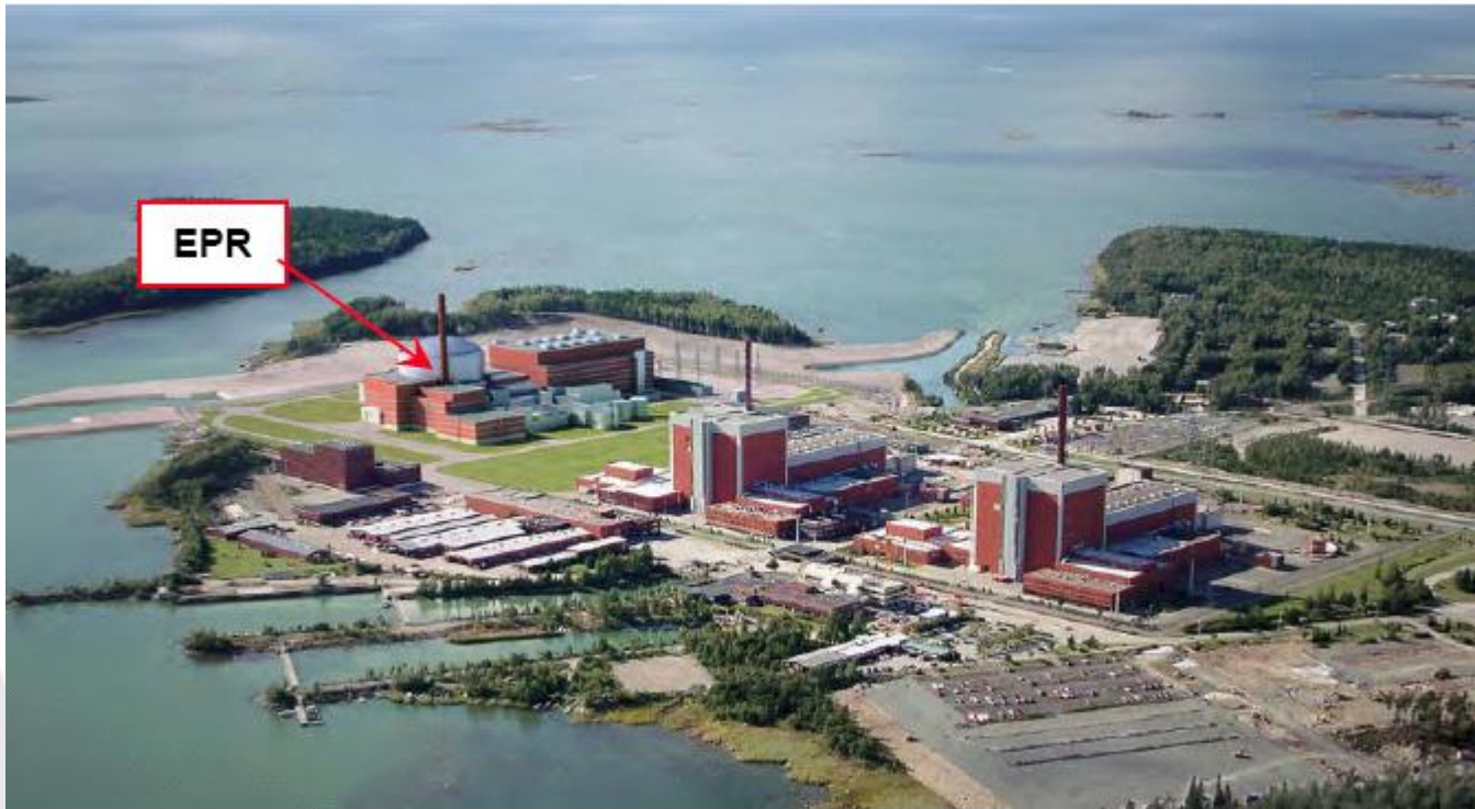
Figure 7 - Artists impression of the completed EPR reactor at Okiluoto
